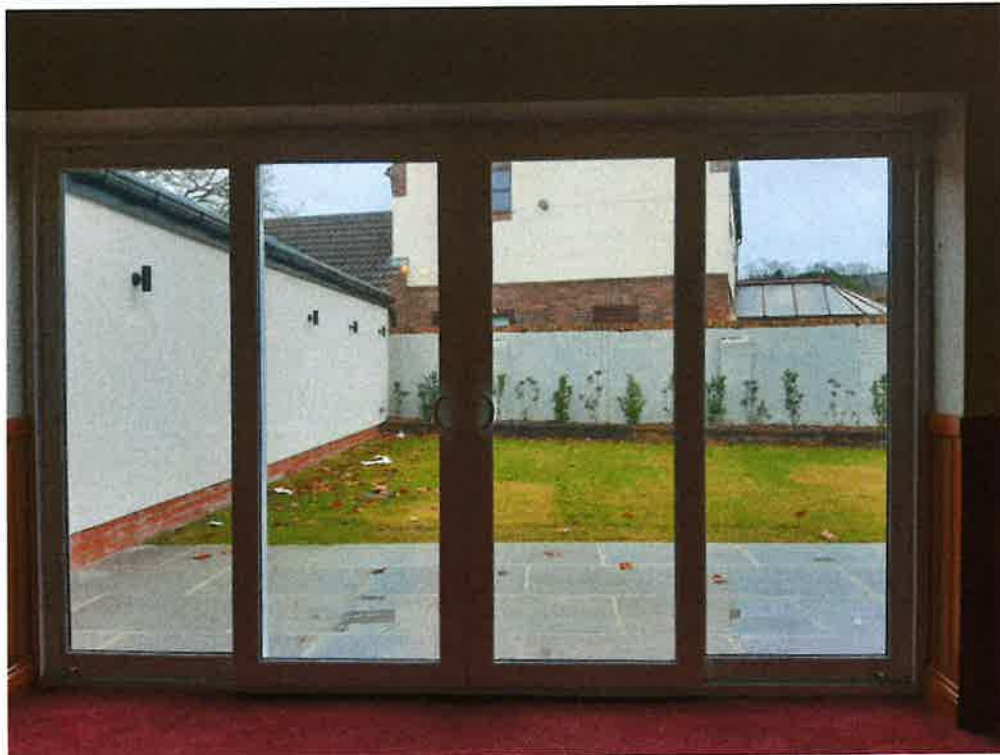
13 View from function room towards the property North of The Comus Inn
